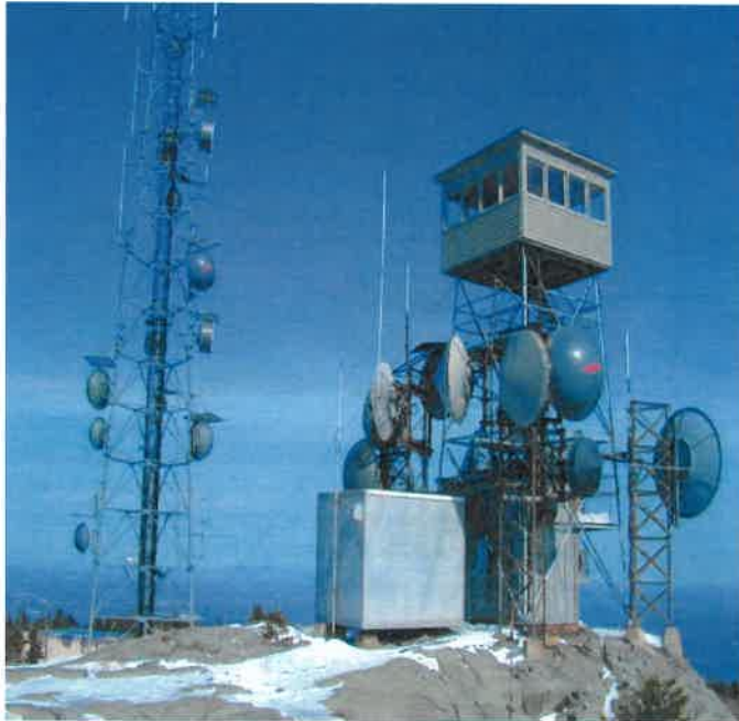
Mt. Kearsarge Communications Tower and Fire Tower
